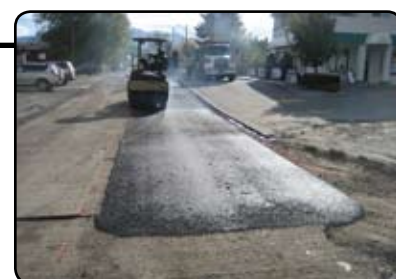
October 6, 2009 Roads Rehabilitation Project begins
