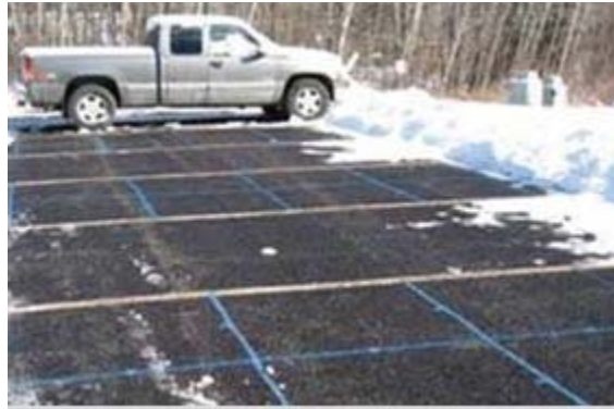
Figure 16. Porous asphalt parking lot one hour after being plowed. Photo courtesy of the University of New Hampshire Stormwater Centre.
