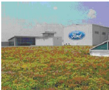
Figure 2. An extensive green roof at the Deerborn Michigan, Ford Assembly Plant. (picture courtesy of Green Roofs for Healthy Cities and William McDonough + Partners, ARCADIS).
