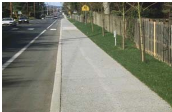
Figure 7. Pervious concrete is used for a sidewalk in Olympia, WA. Photo courtesy of City of Olympia, WA.
