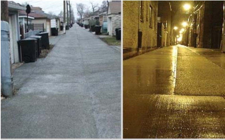
Figure 11. Two of Chicago's Green Alley designs incorporate pervious concrete, a full alley width installation (left) and centre strip of alley installation (right). Photos courtesy of Chicago Department of Transportation.
