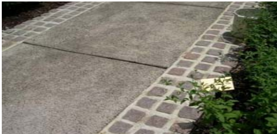
Figure 6. Pervious concrete walkway bordered by paving stones, Washington D.C. Photo courtesy of the Low Impact Development Center Inc.
