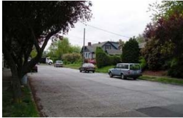
Figure 8. A residential street in Portland, OR uses pervious concrete to reduce combined sewer overflows.. Photo courtesy of Portland Bureau of Environmental Services.
